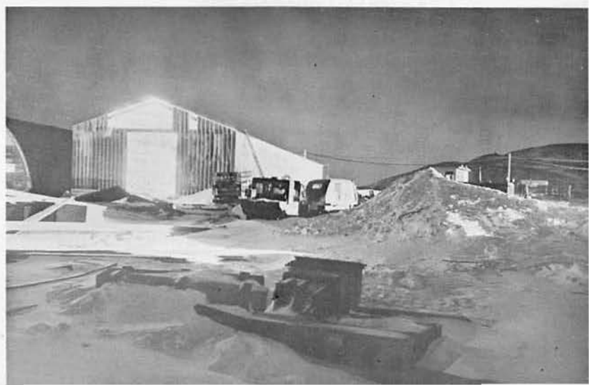
The Public Works garage was completed by flood light.
