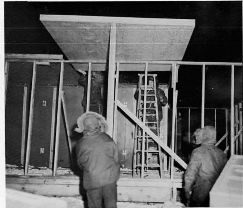
New overhead goes up fast due to prefabricating the roof panels.
