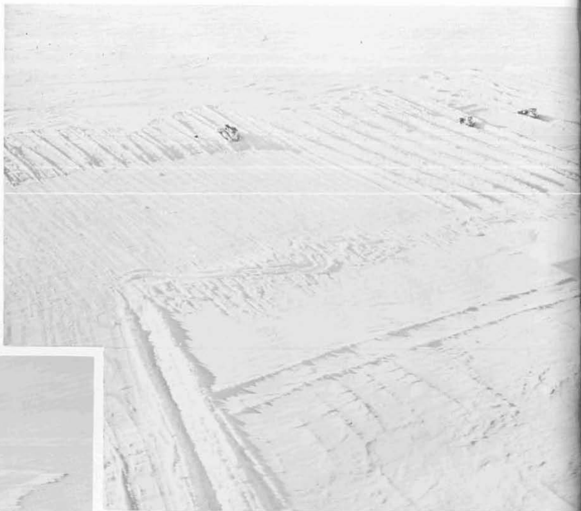
The D-8 cats are almost hidden in the furrows as they push mountains of snow off the runway.
