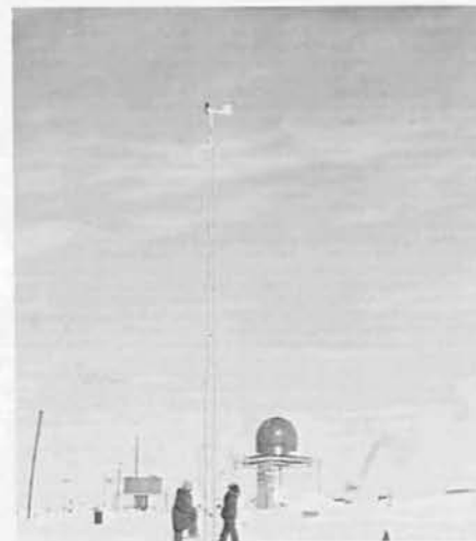
New wind velocity and direction tower is erected by station meteorologists.
