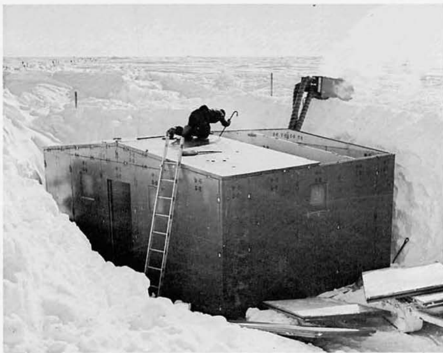
New geo-magnetic building is erected early in the year.
