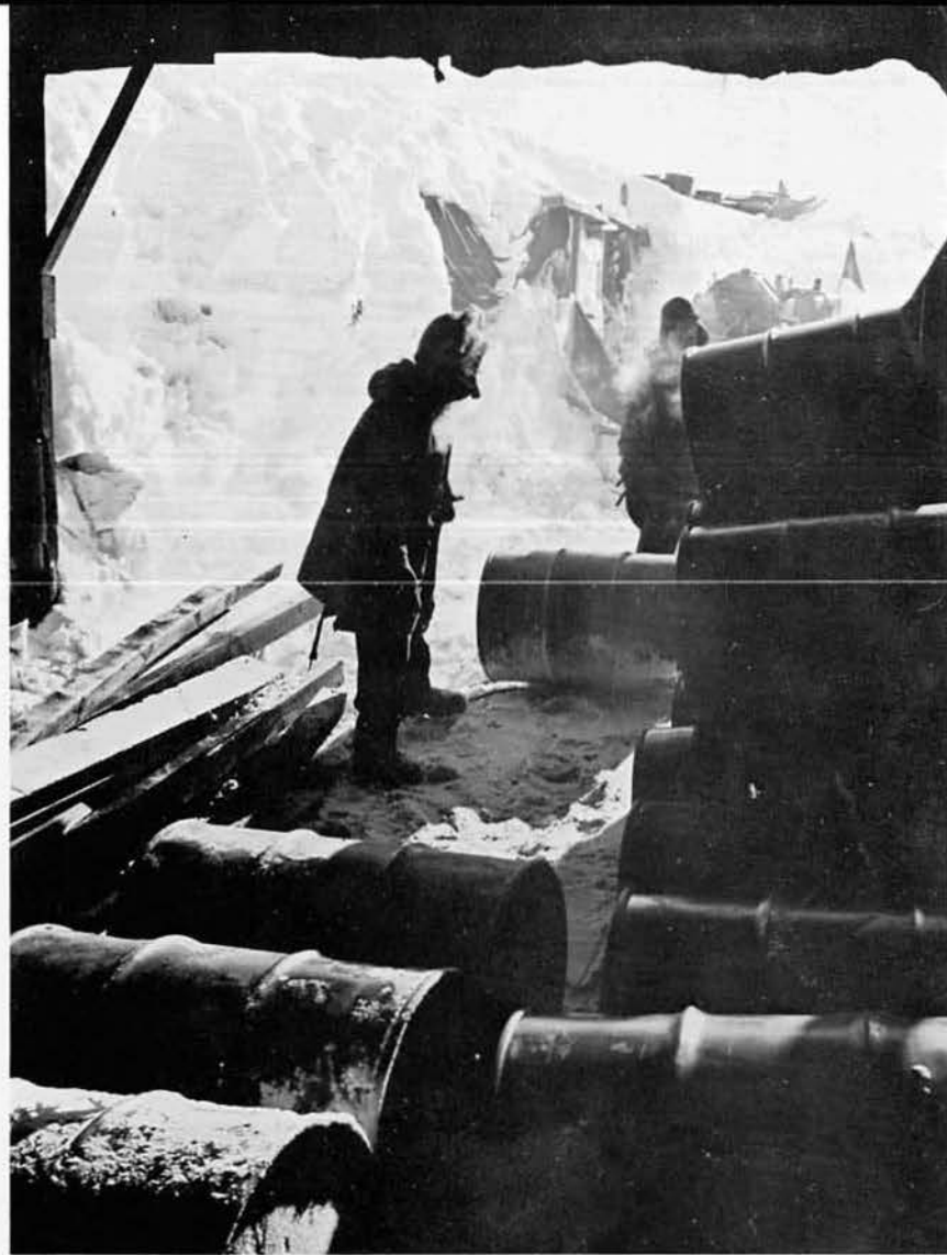
South Pole men stack empty fuel drums for later use as roof supports in passageways between the camp's buildings. Much time was used working on camp maintenance.
