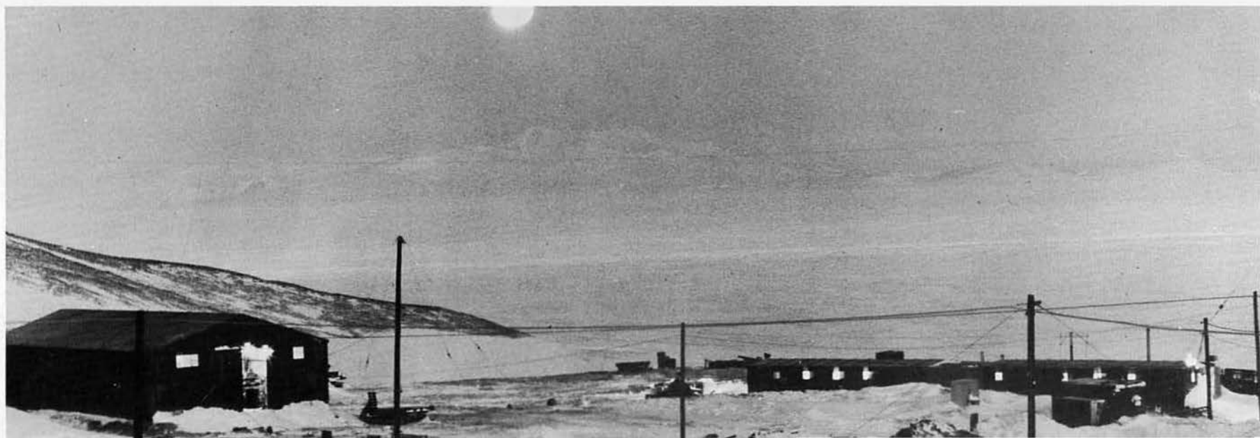
The USARP garage at left, and the new Bio-Lab at right showing the added extension.
