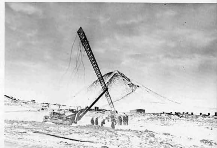
New antennas were raised.
