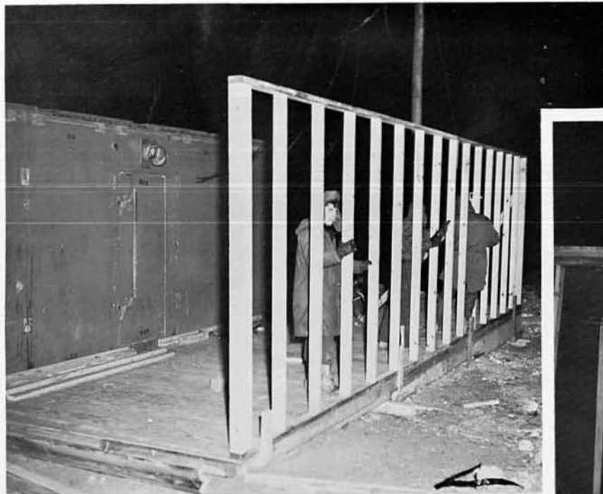
Wall on extension goes up
