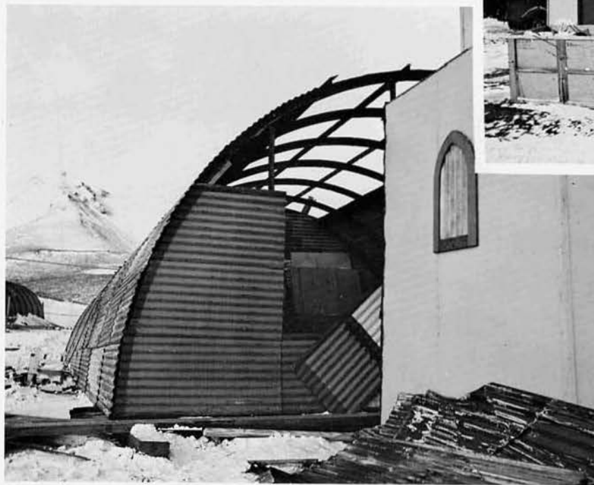
A Chapel extension was built....
