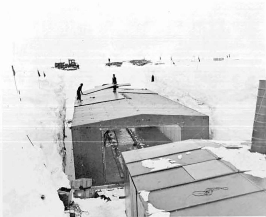
Finishing touches being put on new garage, new powerhouse in foreground.
