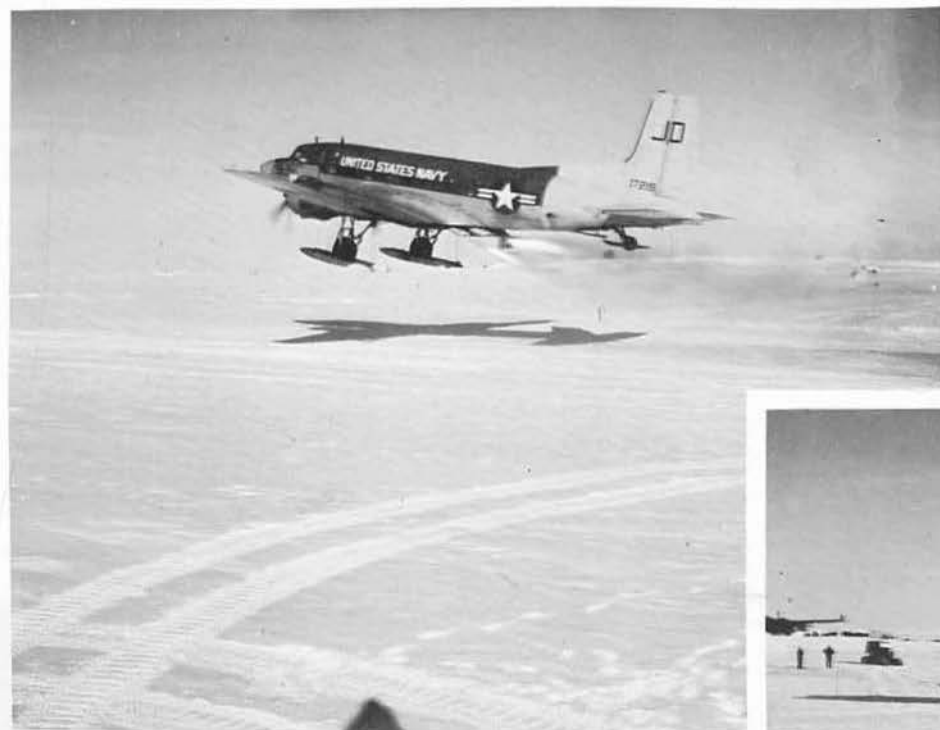
The R4D used Jato assist whenever taking off with full load
